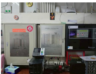
Fire Alarm Control Panel
